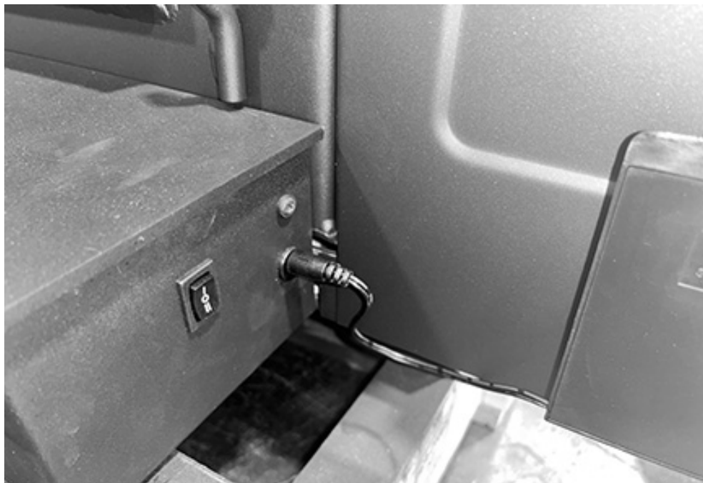
Figure 22: Battery box plugged in.
