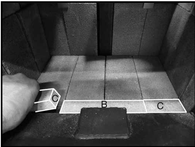
Figure 30: Narrow front bricks in place.
