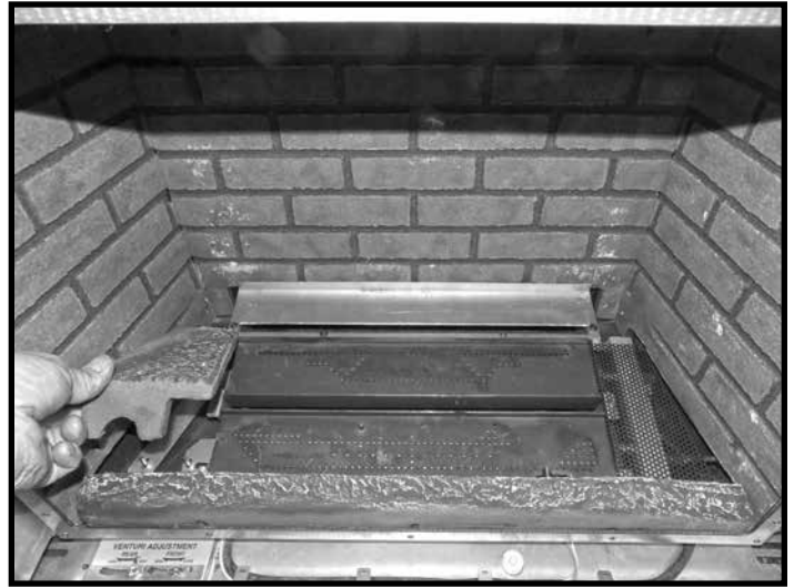
Figure 68: Installing left side base piece.
