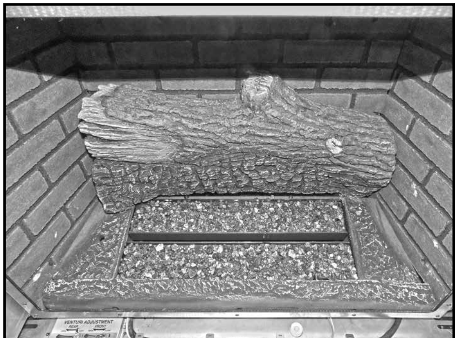
Figure 74: Ember pieces spread on top of burner trays.
