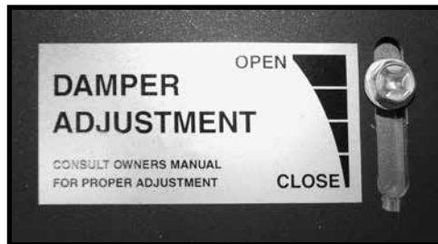
Figure 43: Damper adjustment indicator.
