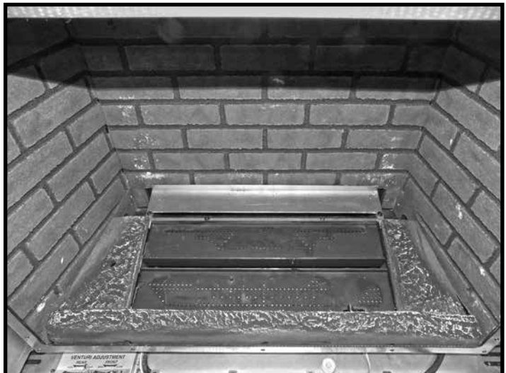
Figure 70: All three base pieces in place.
