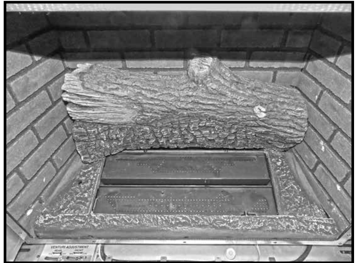
Figure 72: 1st log placement.
