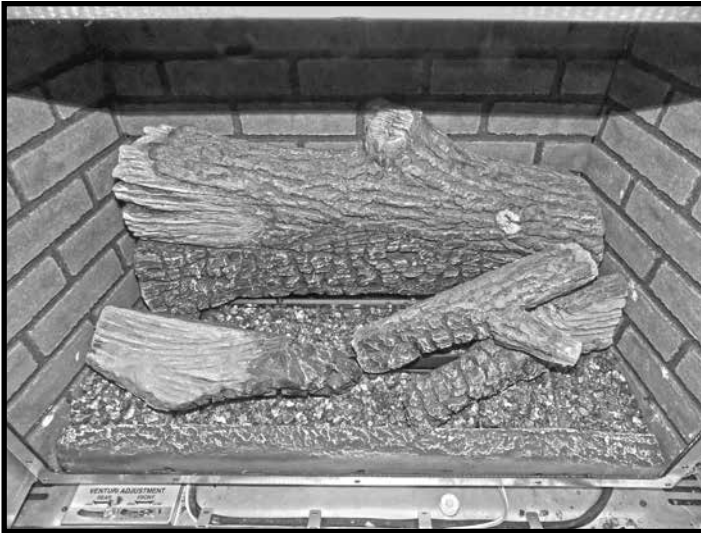
Figure 79: 4th log placement.
