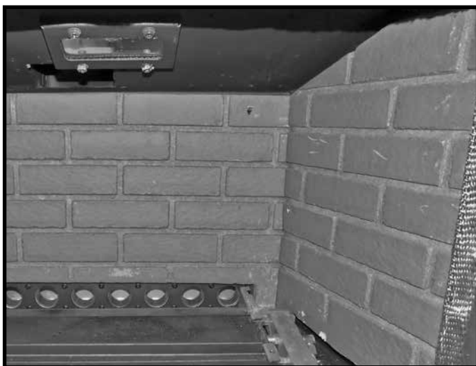
Figure 26: Right side panel in place.
