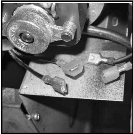
Figure 15: Disconnecting fan wires.
